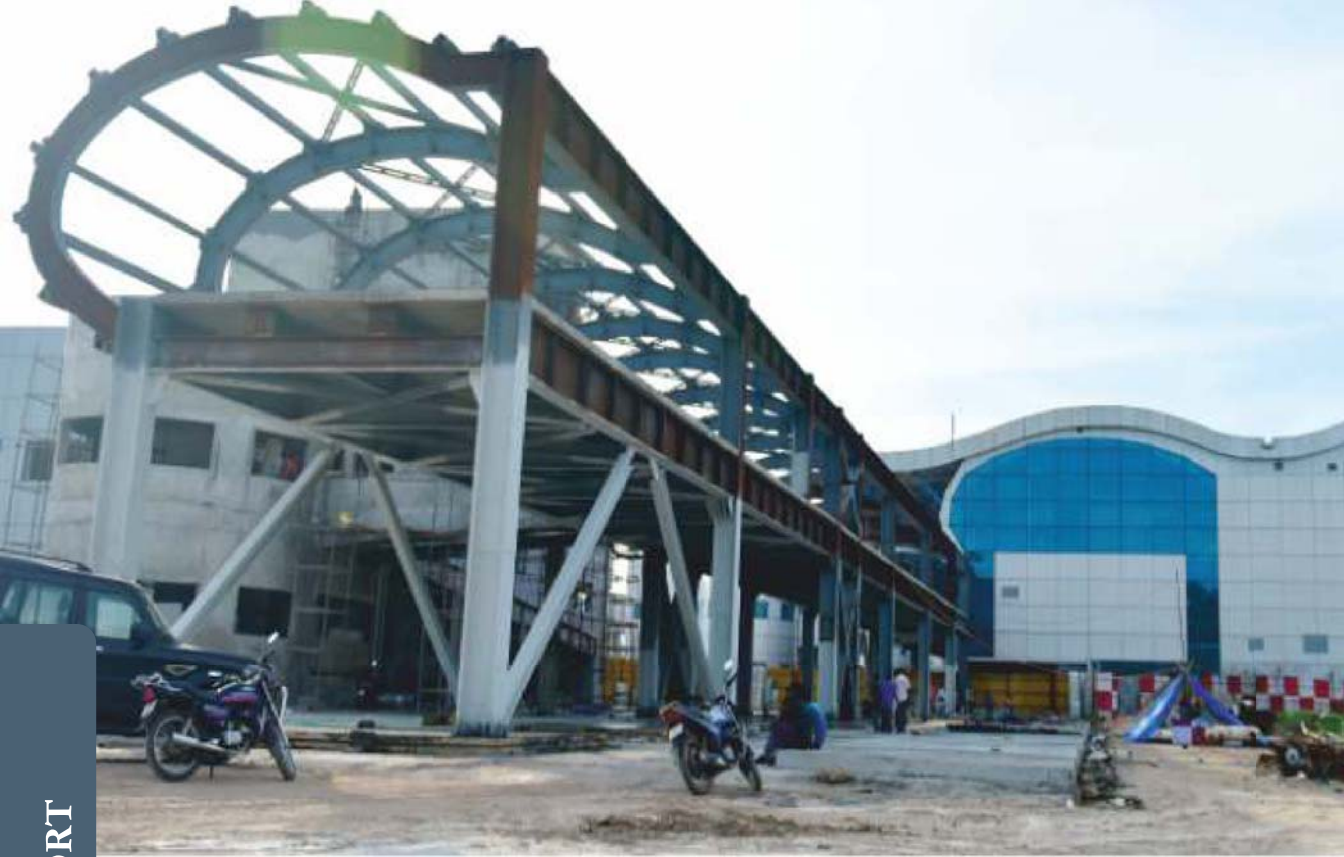
fourth aerobridge under construction in Trivandrum International Airport.
