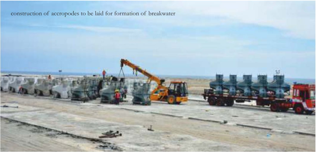
Piling in progress
