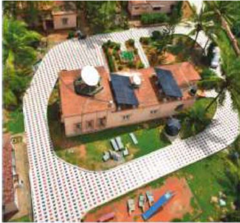
Interlocking Tiles Laid ( Ariel View )
